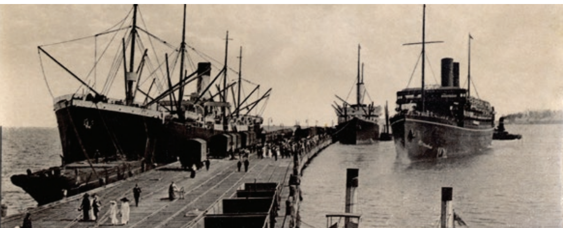
Station Pier, 1901 - 1911. pm1972
